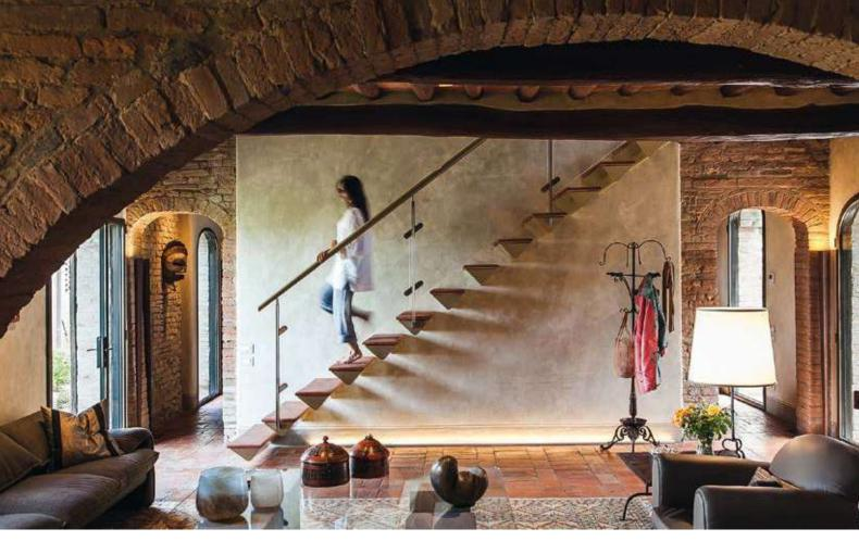
The impressive, entirely cantilevered staircase, might be called a feat of engineering. Fulvio Di Rosa told us about the steel beam hidden by the plastered wall, the three rolled bars supporting each step, about anchoring them to the floor, and about the pilasters that enabled
